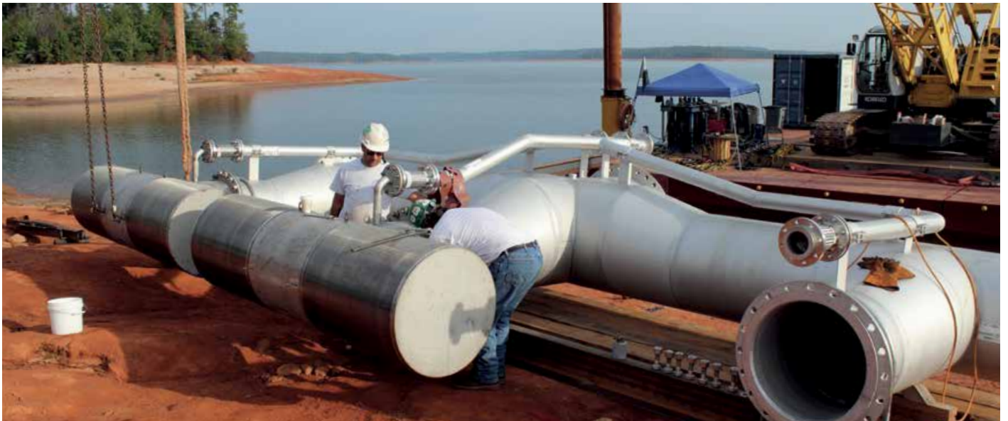
Installation eines Johnson Offshore Intake Systems™: Trinkwasseranlage in South Carolina, USA
