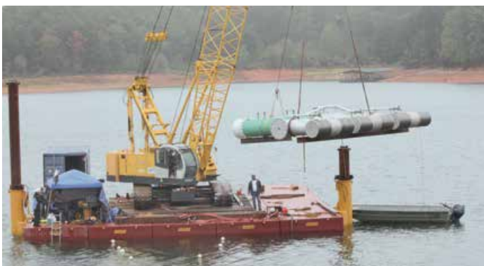
Installation eines Johnson Offshore Intake Systems™ (JOIS™)
