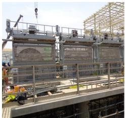
**Figure 4.** Desalination Plant, Barka 4 IWP, Oman. 3 x Zero-Carryover through flow machines (by Aqseptence Group, called MultiDisc) in combination with Cable-Operated Bar Screens 13,600 m<sup>3</sup>/h per channel; material of construction is mainly Duplex combined with a with impressed current cathodic protection
