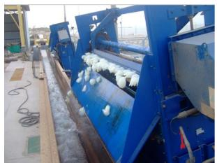
**Figure 3.** Power and MSF-Desalination Plant - Qurrayah, Kingdom of Saudi Arabia. Upgrading with 20 Revolving Chain Screens (by Aqseptence Group), thus removing up to 60 t/h jellyfish per machine out of sea at a total flowrate of 700,000 m3/h; material of construction of submerged parts is 316L with impressed current cathodic protection
